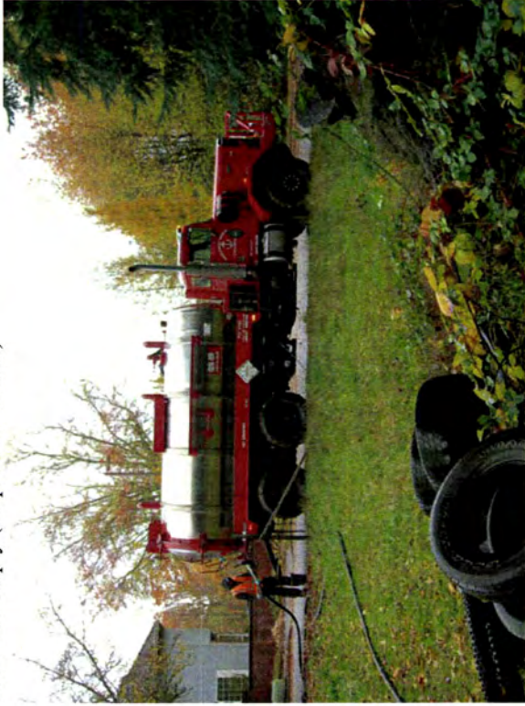
Rinsing interior of tank prior to removal
